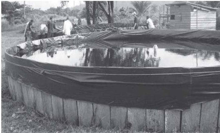
Figure 7: Circular holding tanks
