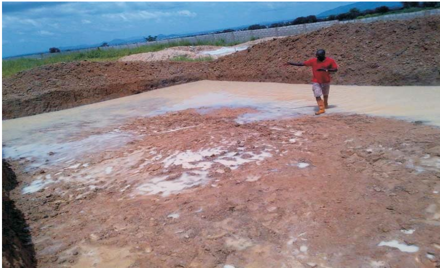
Figure14: Constructing earthen fish pond
