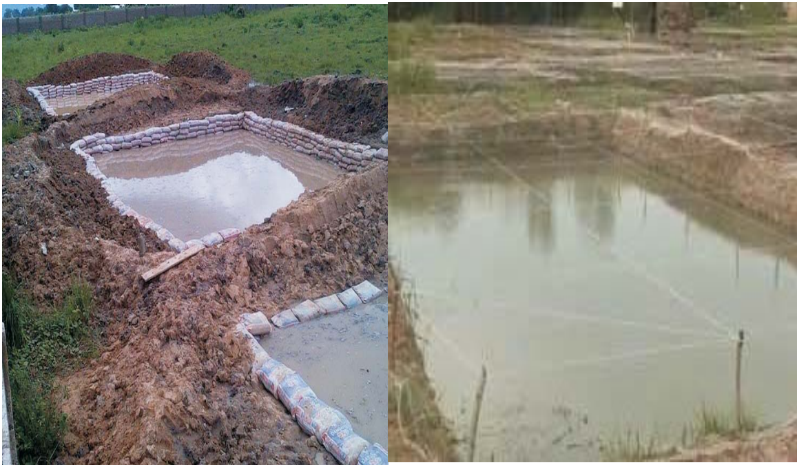
Figure 17 An excavated Fish Pond
