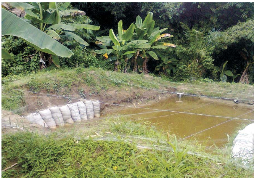
Figure 23 Sand Bagging and Wire Mesh fencing that is expected to prevent flood
