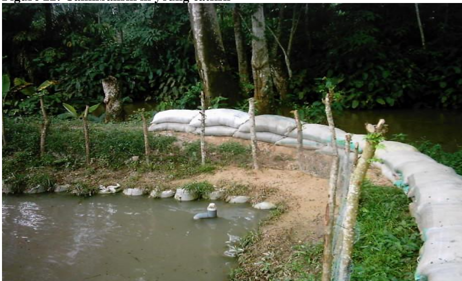
Figure 23: Sand Bagging and Wire Mesh fencing that is expected to prevent flood
